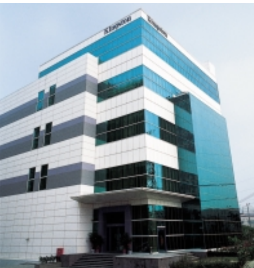
KINGSTON TECHNOLOGY FAR EAST ESTABLISHED MANUFACTURING IN TAIWAN IN 1997. PHOTO DEPICTS THE NEW FACILITY IN HSIN-CHU BUSINESS PARK OPENED NOVEMBER 2000.
